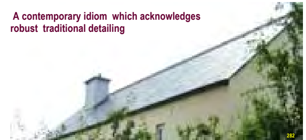
Flush verge, plaster eaves and rainwater gutter same colour as roof
