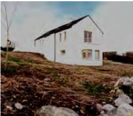
Narrow plan - slope can adapt and absorb the slope into the design - reducing sitework costs
